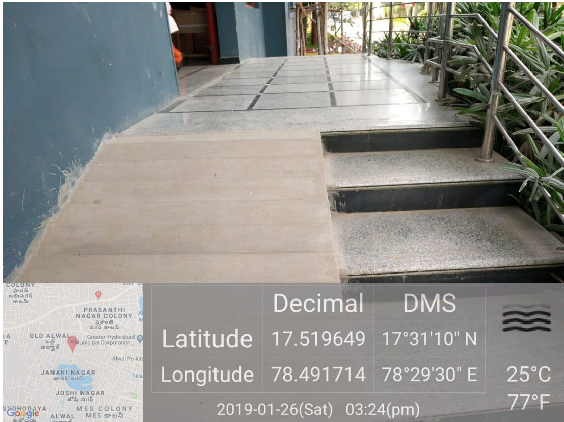
Ramp at the Entrance of M.V Block
