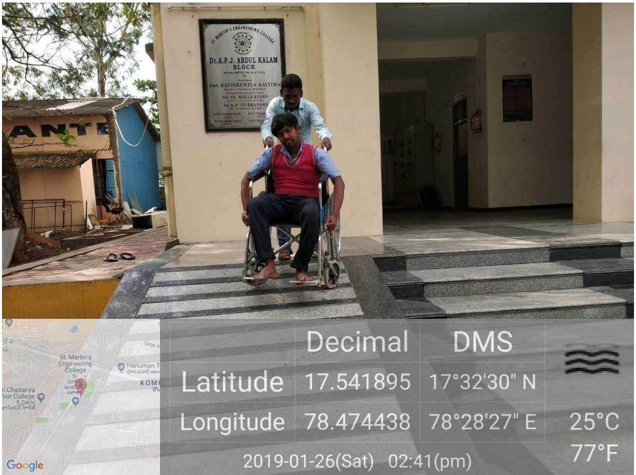
Ramp at the entrance of Training & Placement Wing
